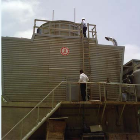
Project : Internation Steel Limited LHC-373D-C1, 44-32-29 °C, 180 M 3 /Hr./Set
