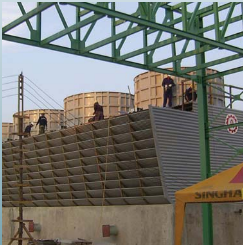
Project : Rajburi Ethanol Plant LHC-458D-C4, 42-34-29.4 °C, 700 M 3 /Hr./Set
