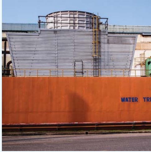
Project : Thai Cold Rolled Steel Sheet Public Company Limited LHC-475D-C4 37-32-28 °C 2,800 M 3 /Hr./Set
