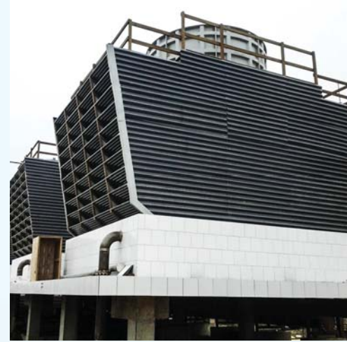
Project : Ibrahim Fibre Power Plant (Phase III) LHC-452D-C1x 5 Sets, 50-34-30 °C, 250 M 3 /Hr./Set
