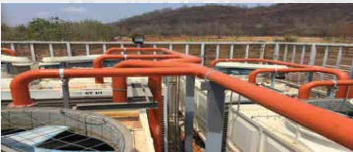
LOCATION : GOVERNMENT PHARMACEUTICAL ORGANIZATION MODEL : FRP COOLING PIPE COATING 230 M2 THINKNESS 3 mm.
