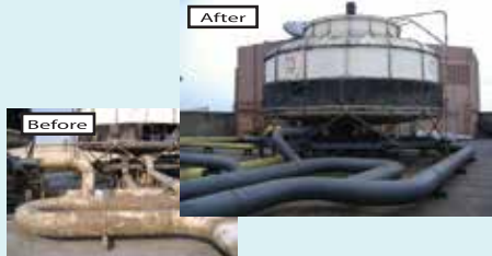
LOCATION : LE CONCORDE, BANGKOK MODEL : F.R.P. LINING PIPE AND SUPPORT 260 m 3
